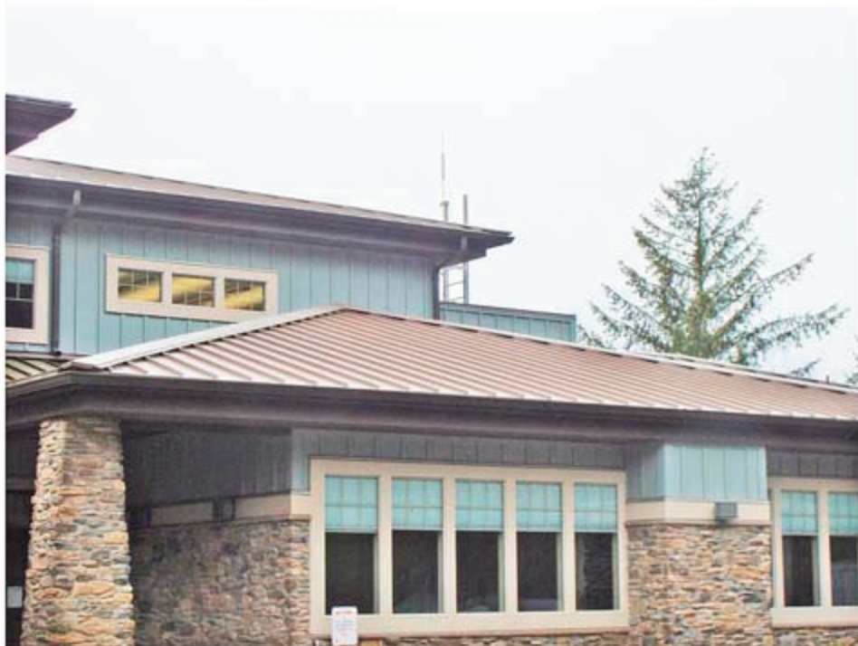
The antenna is easily seen from the parking lot. Looks like it belongs there?
